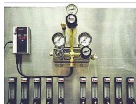
**Figure 4. Point of use panel that regulates process gas pressure and flow.**
