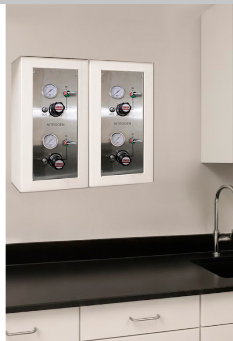
casework installation shown
